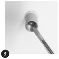
Mount suspension kit body on to the ceiling.
